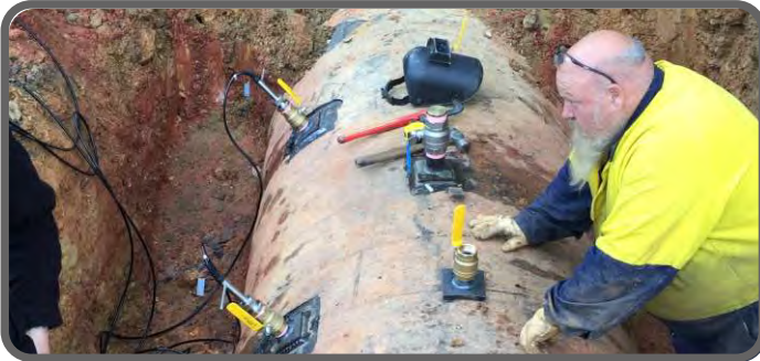
DN800 Water Supply
