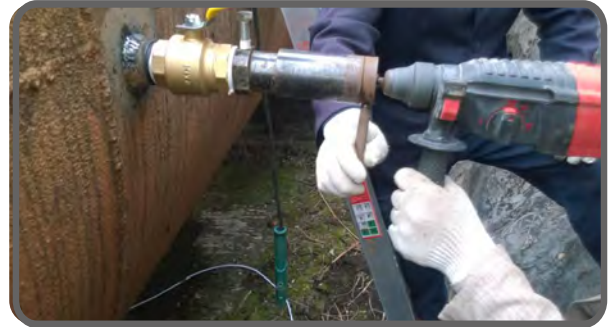
Insertion Transducer Installation
